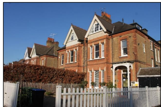
Fig. 56. 108 to 114 Ravensbourne Avenue, west elevations
