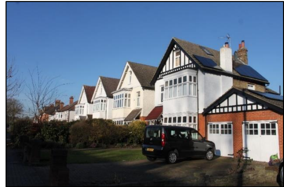
Fig. 55. 88 to 94 Ravensbourne Avenue, west elevations
