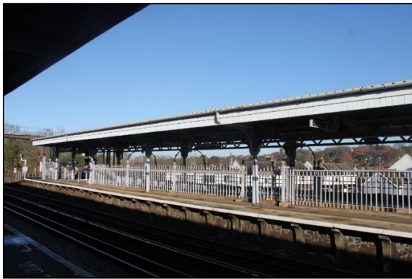
Fig. 23. Station platform, looking east
