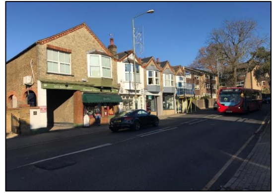
Fig. 31. 34 to 42 Beckenham Lane, south elevation
