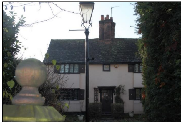
Fig. 13. The Old Cottage, north-east elevation
