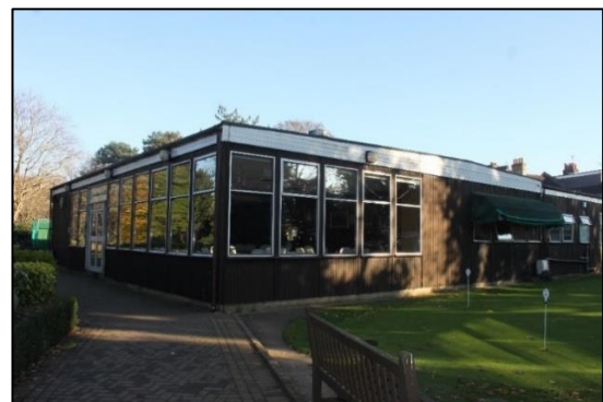
Fig. 57. The Shortlands Golf Club clubhouse, north and west elevations
