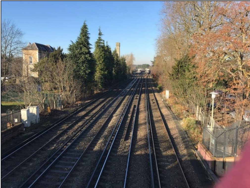
Fig. 5. View from pedestrian bridge at Queens Mead, looking north
