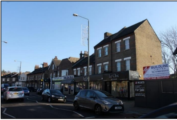
Fig. 28. 75 to 85 Beckenham Lane, north elevations
