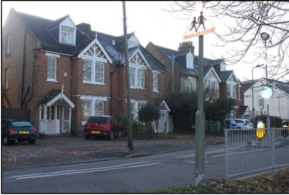
Fig. 46. 35 to 41 Queens Mead, north elevations
