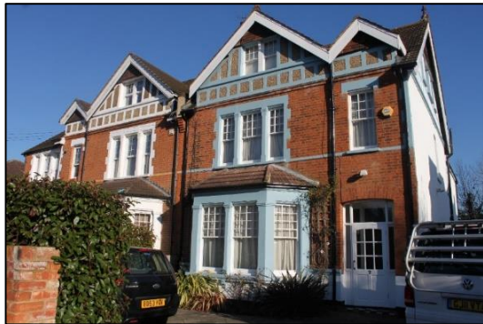
Fig. 16. 5 & 7 Valley Road, west elevation
