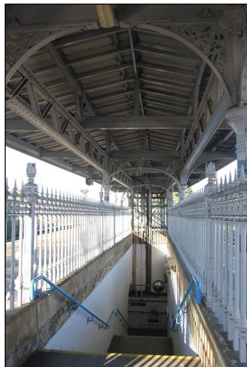
Fig. 21. Station platform, ironwork
