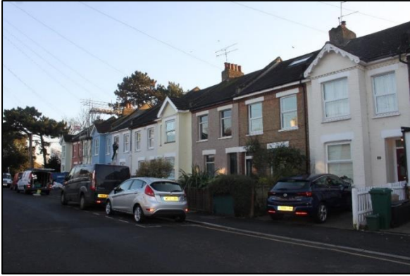
Fig. 40. 33 to 13 Martin's Road, north west elevations
