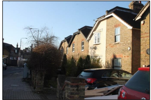
Fig. 33. 60 to 78 Beckenham Lane
