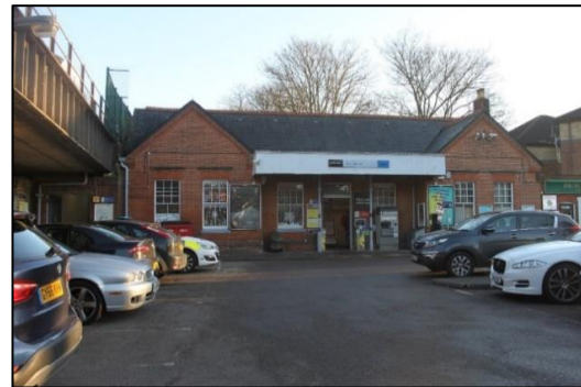
Fig. 20. The Station and forecourt, north elevation
