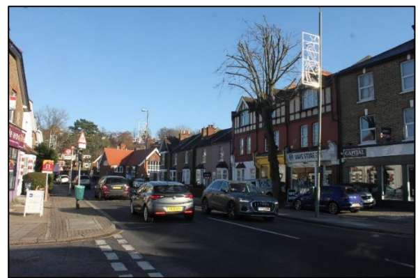
Fig. 26. 39 to 55 Beckenham Lane, north elevations
