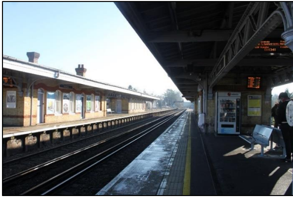
Fig. 22. Station platform, looking south
