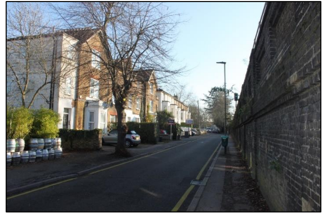
Fig. 37. 1 to 10 Station Road, west elevations
