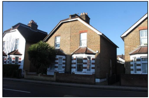
Fig. 32. 48 and 50 Beckenham Lane
